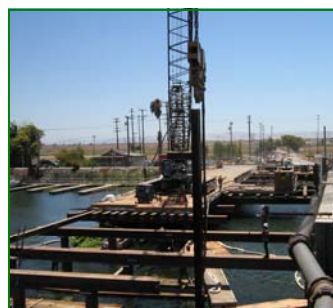
Crews working on the southern temporary trestle
