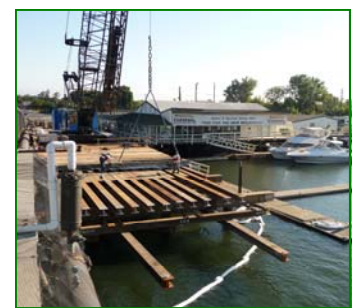
Dropping the decking for the temporary trestle at the northern levee
