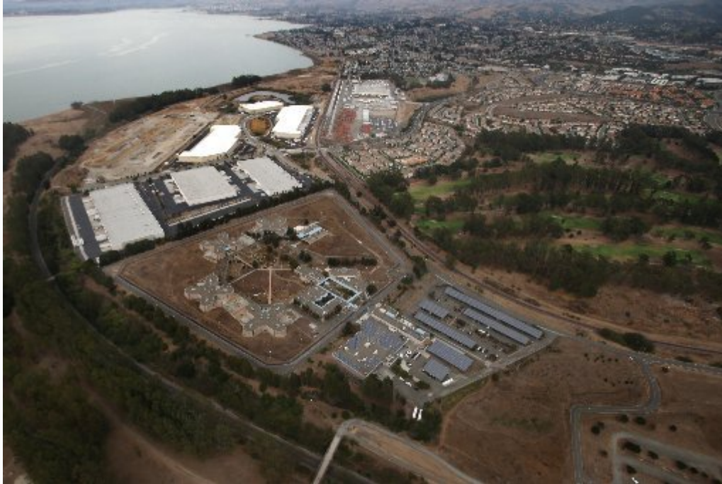
Aerial shot of the West County Detention Facility. File photo nu Ray Chavez
