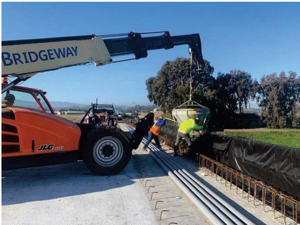
Figure 3 – Pouring Exterior Shear Keys
