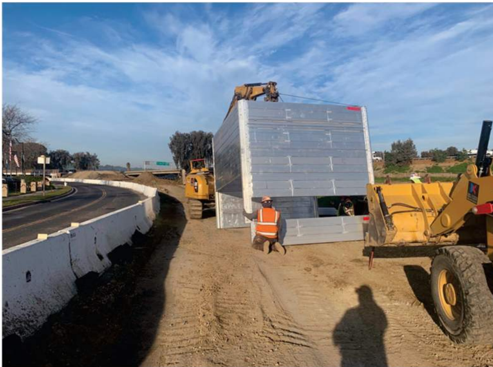
Figure 2 – Drainage System 2 – Temporary Shoring System
