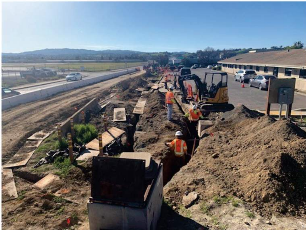
Figure 3 – AT&T 5000 Marsh Service Relocation
