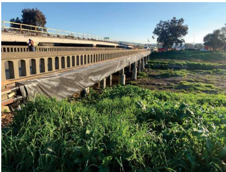
Figure 2 – Existing Bridge Bird Nesting Exclusion System
