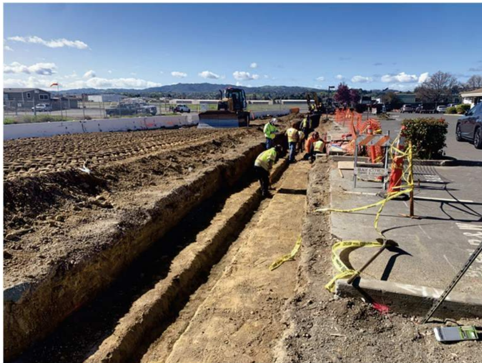
Figure 2 – Retaining Wall Excavation
