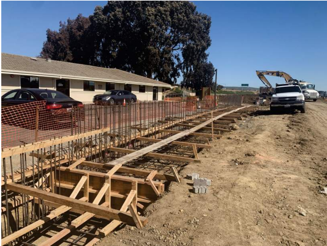
Figure 3 – Retaining Wall Footing Reinforcement
