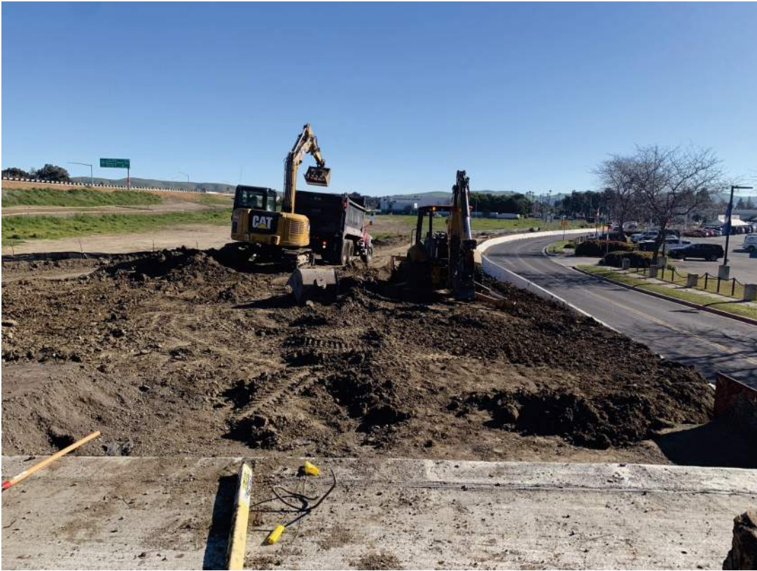
Figure 4 – East Approach Grading
