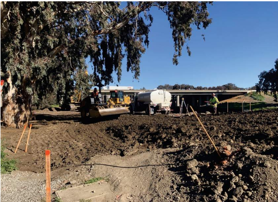
Figure 5 – Access Road 2 Grading
