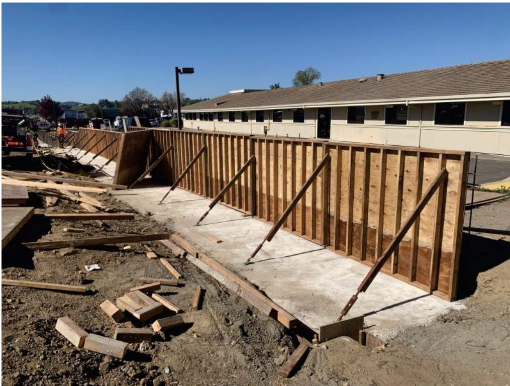
Figure 3 – Retaining Wall Forming
