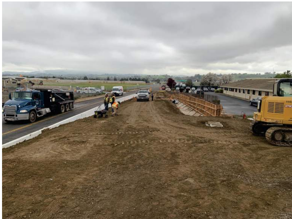
Figure 2 – Retaining Wall & West Approach
