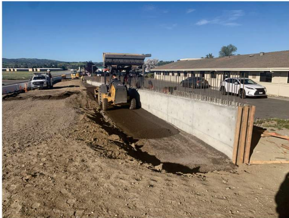
Figure 2 – Retaining Wall & West Approach
