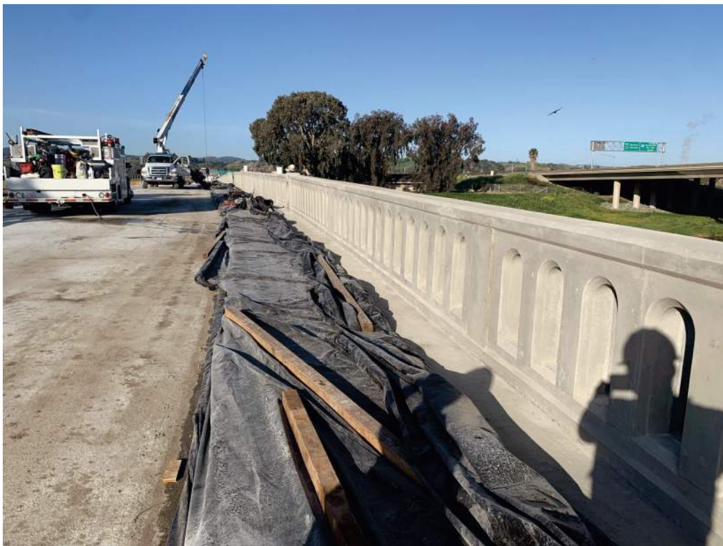
Figure 3 – Concrete Bridge Railing
