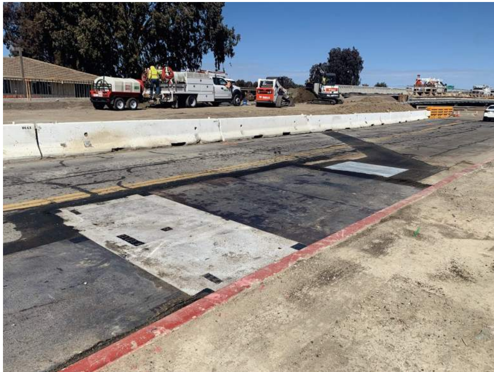
Figure 2 – West Approach & PG&E Vault
