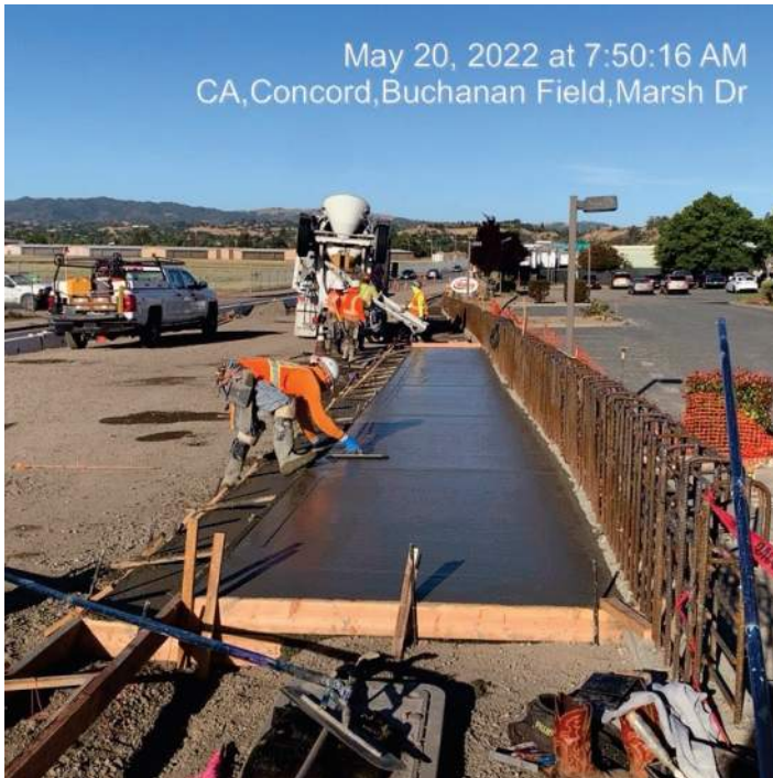
Figure 5 – Curb/ Gutter & Sidewalk at Retaining Wall 1
