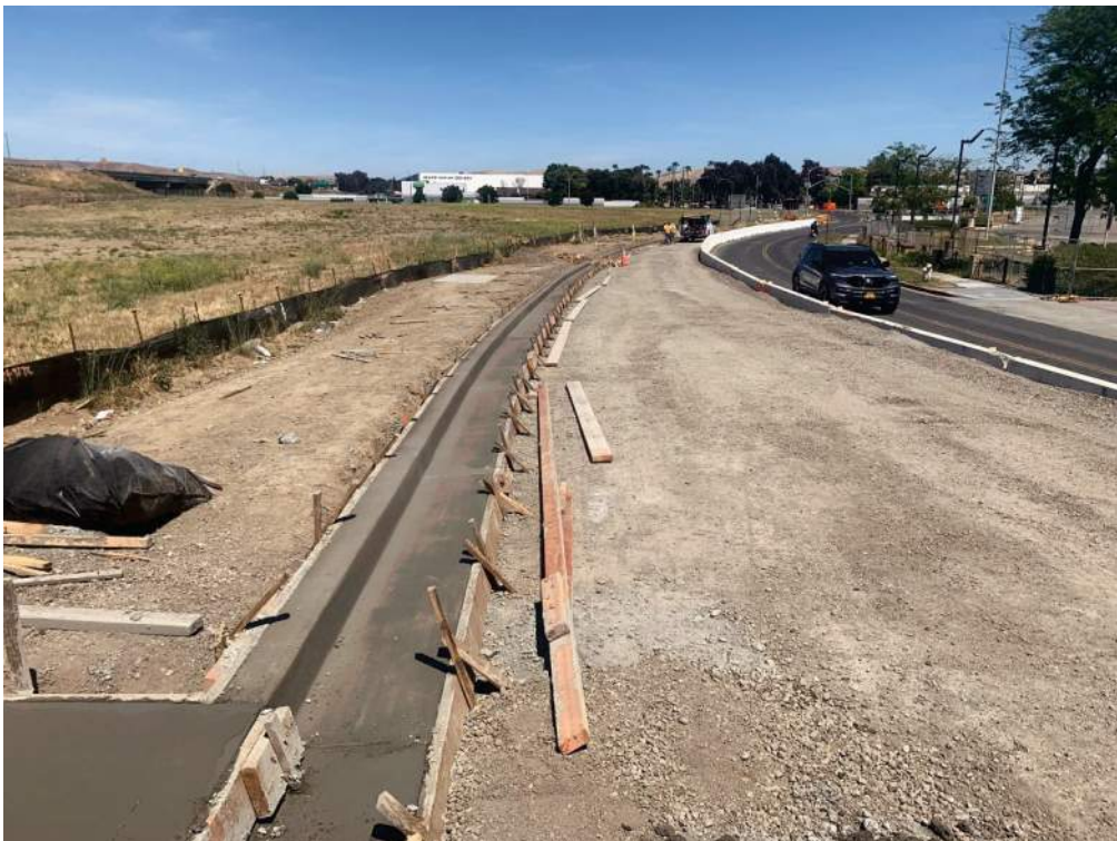
Figure 4 – Curb and Gutter Eastside of Bridge
