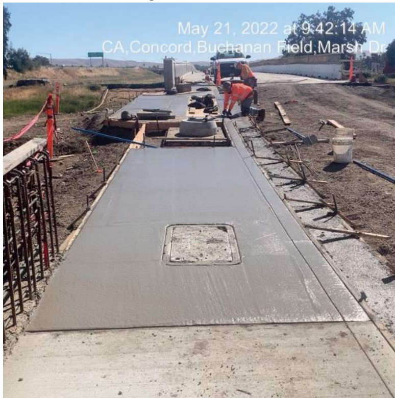
Figure 6 – Access Road 2 Driveway and Sidewalk (Westside of Bridge)
