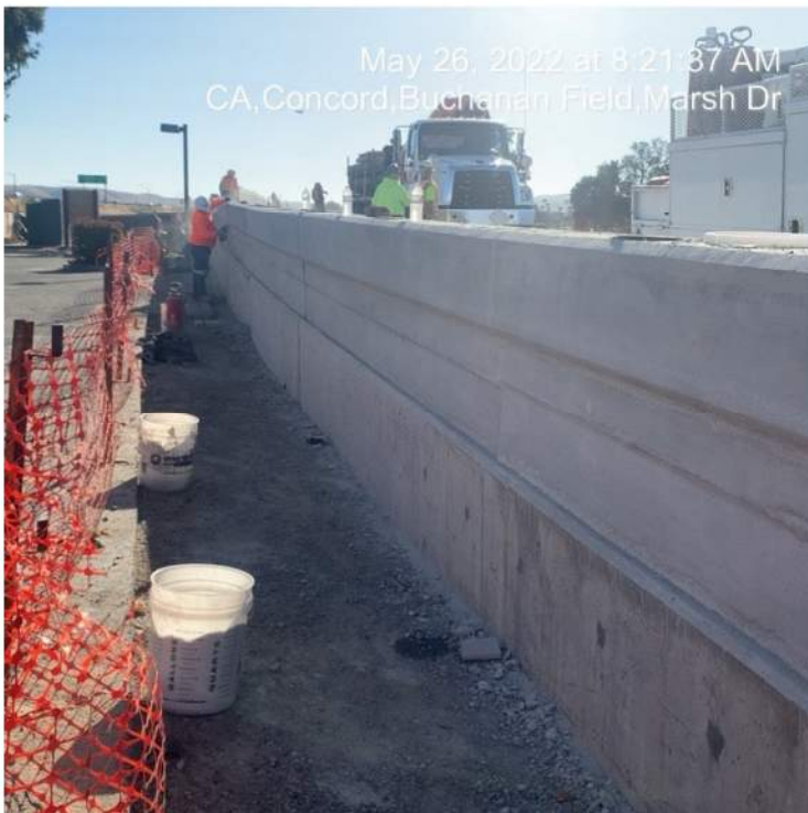
Figure 4 – Concrete Finishing Barrier Rail
