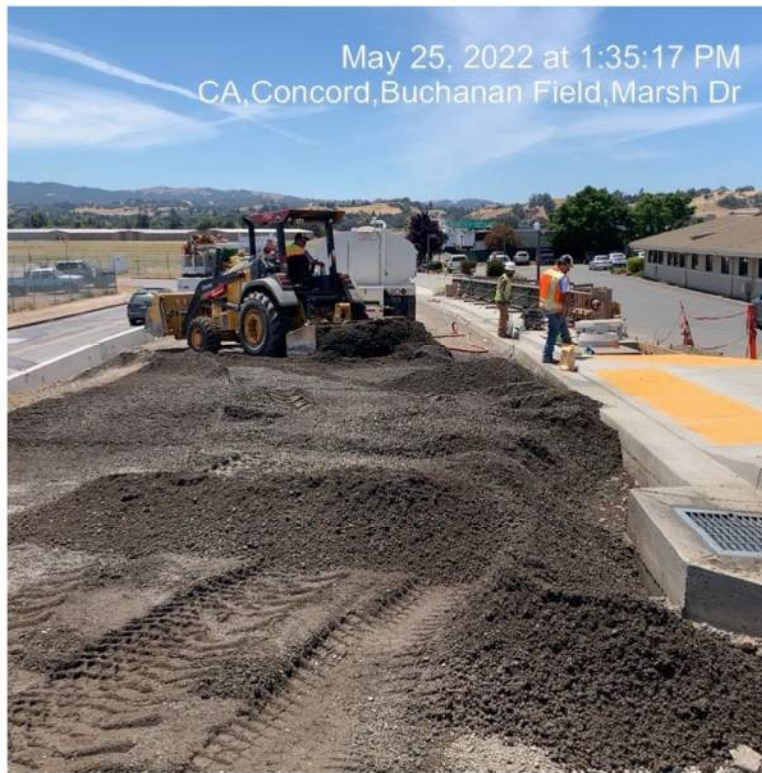
Figure 3 – Class 2 AB Final Lift
