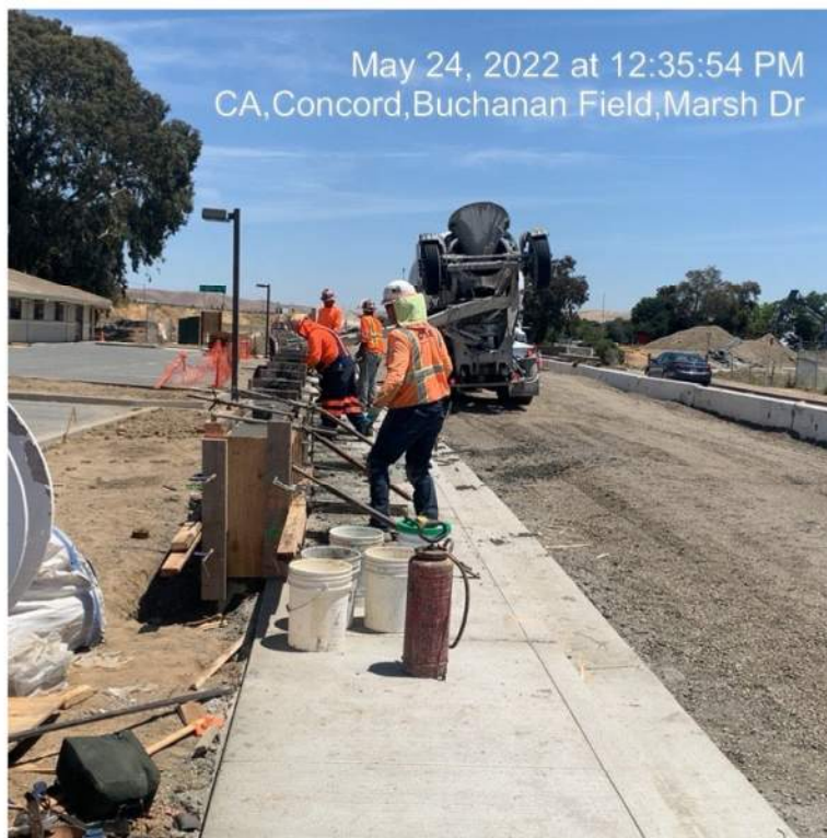
Figure 6 – Concrete Pour – Type 732 Concrete Barrier Rail
