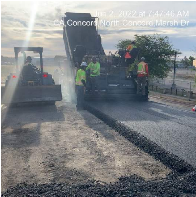
Figure 3 – Stage 1 HMA Paving (Eastside)
