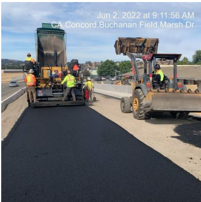
Figure 4 – Stage 1 HMA Paving (Westside)
