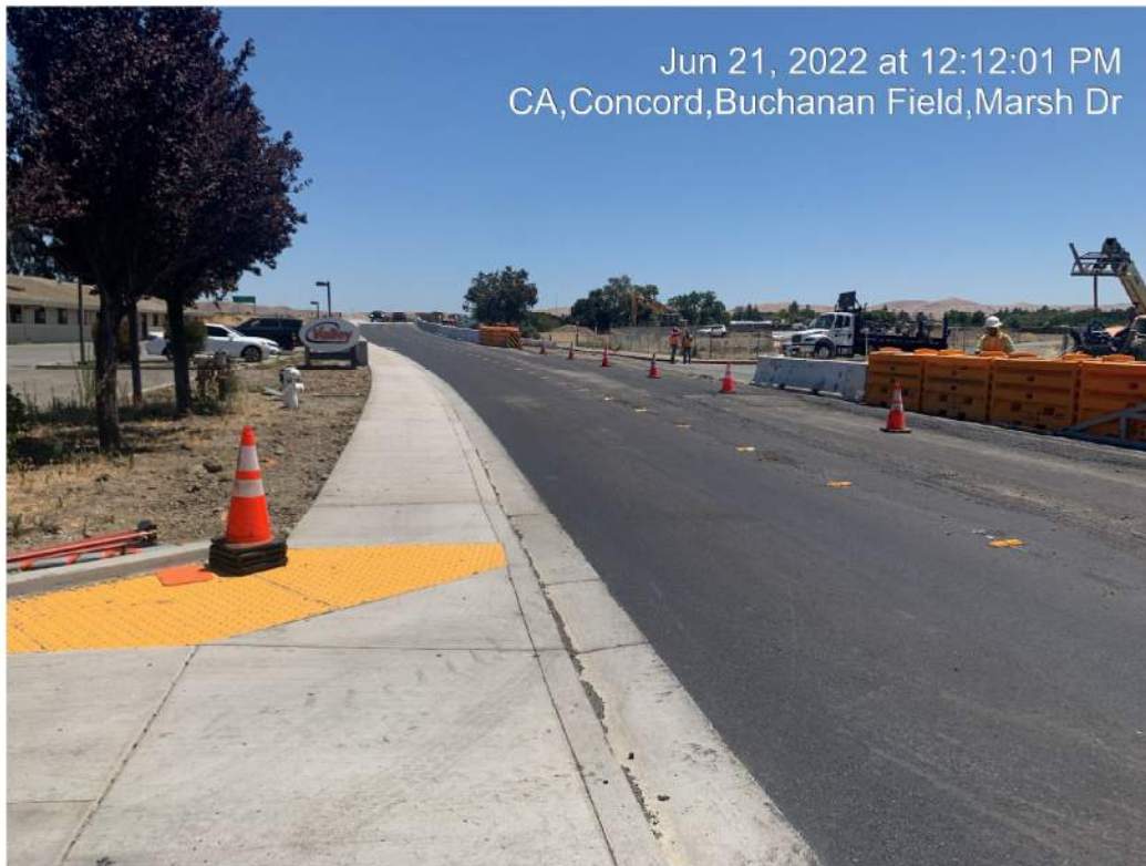
Figure 2 – Stage 2 Traffic Switch
