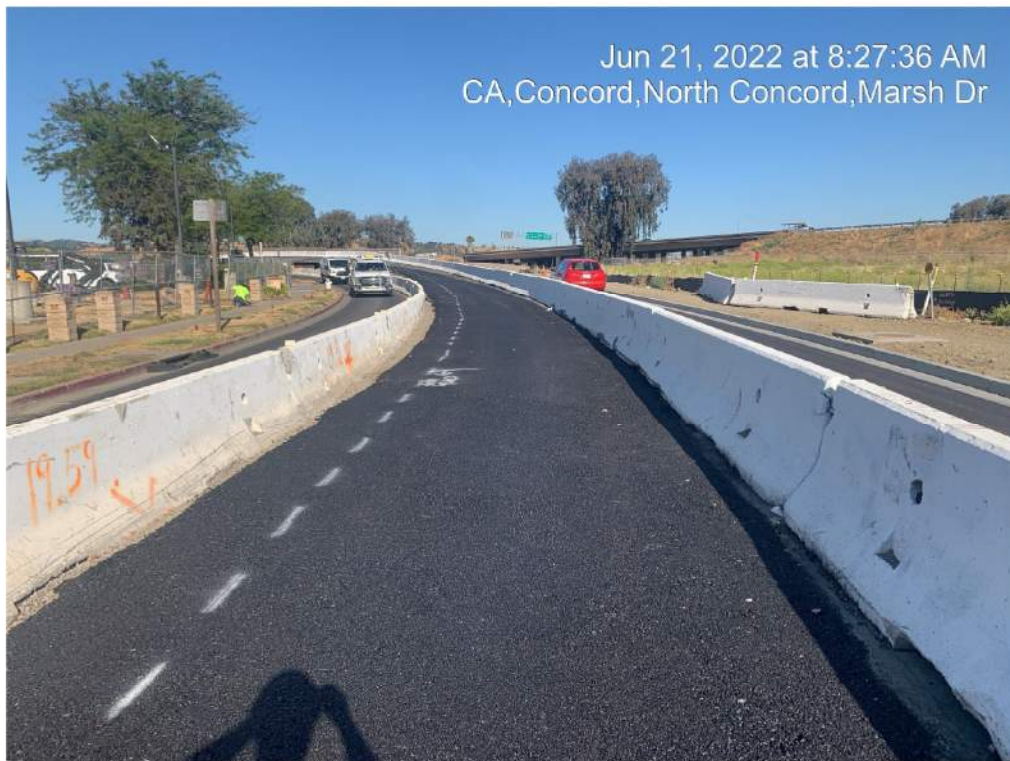
Figure 4 – Stage 1A Road Work
