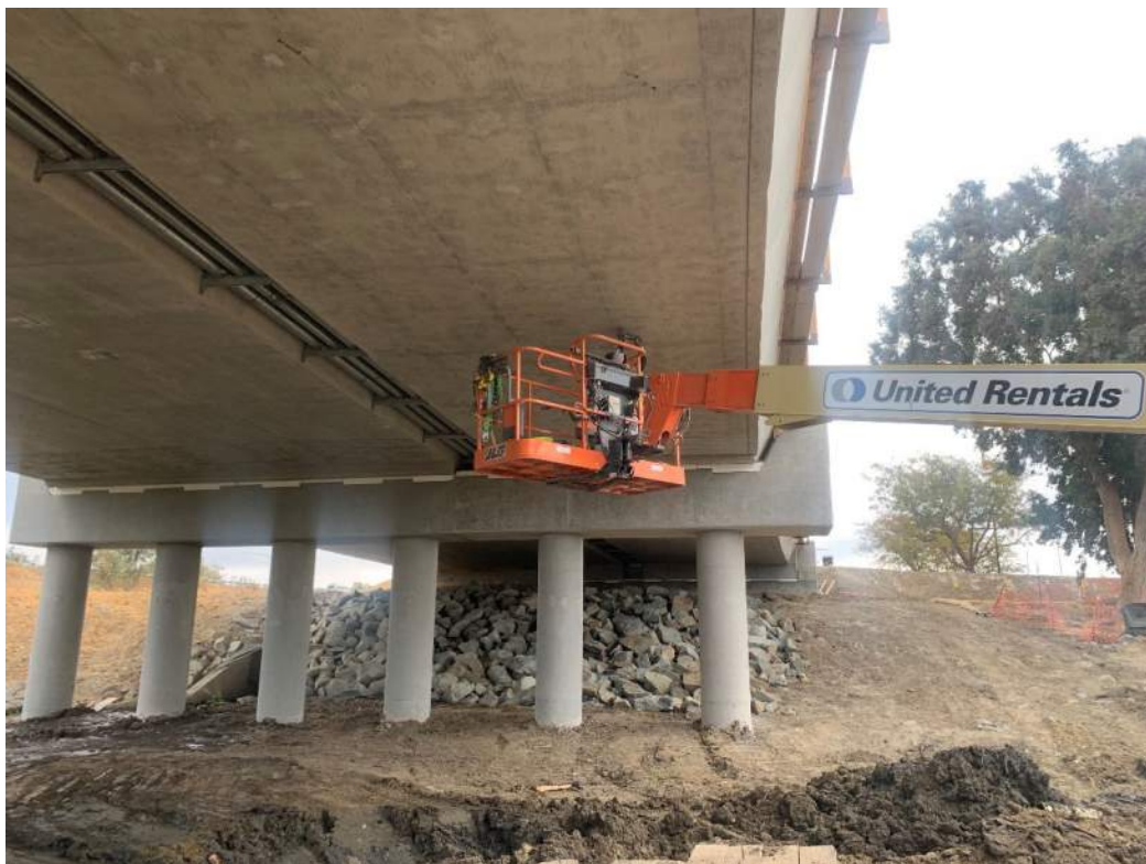
Figure 3 – Concrete Dry Finishing
