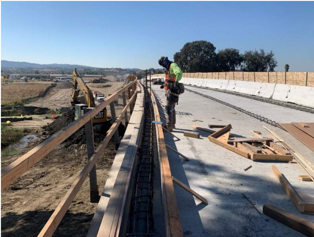
Figure 4 – Form/ Rebar PCC Pedestrian Rail Curb
