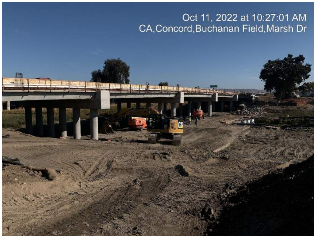
Figure 5 – Bridge Work - Cleanup
