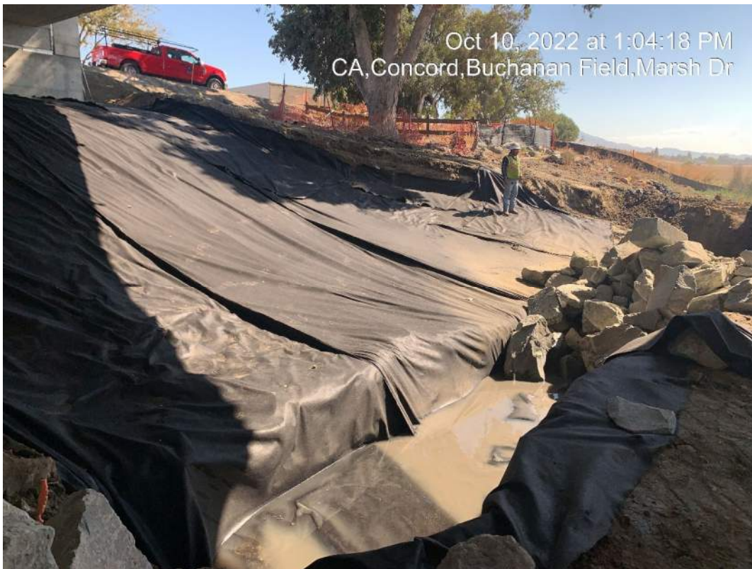
Figure 6 – Rock Slope Protection – Abutment 6
