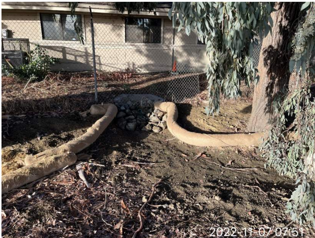
Figure 3 – BMPs Around 5000 Marsh Drive
