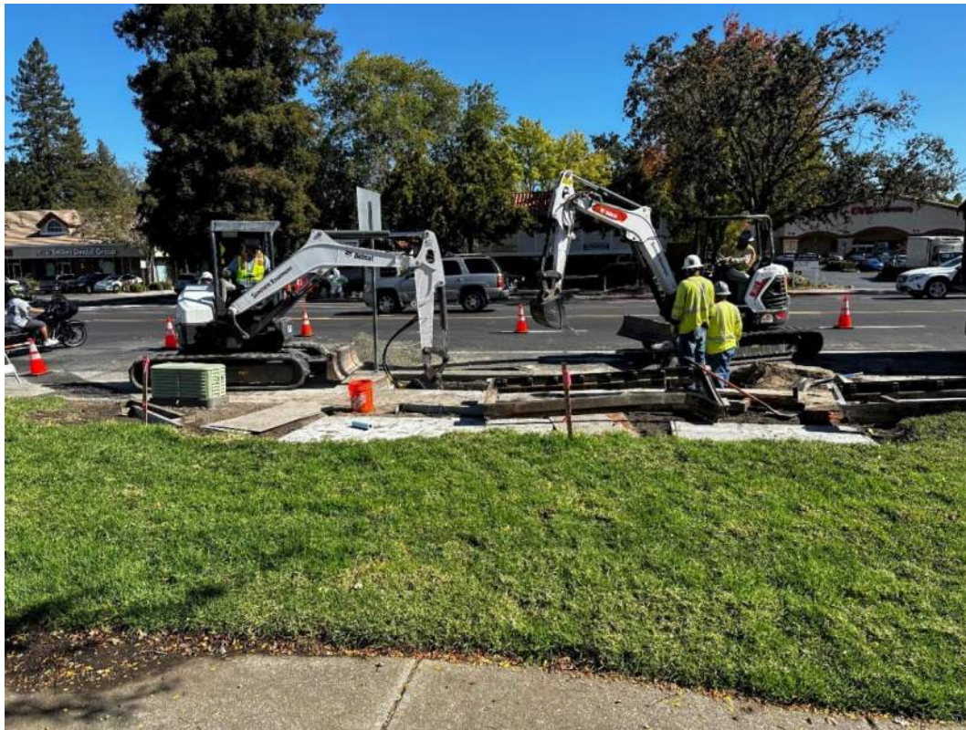
Figure 2. PG&E Electrical Relocation Work completed Fall 2022.
