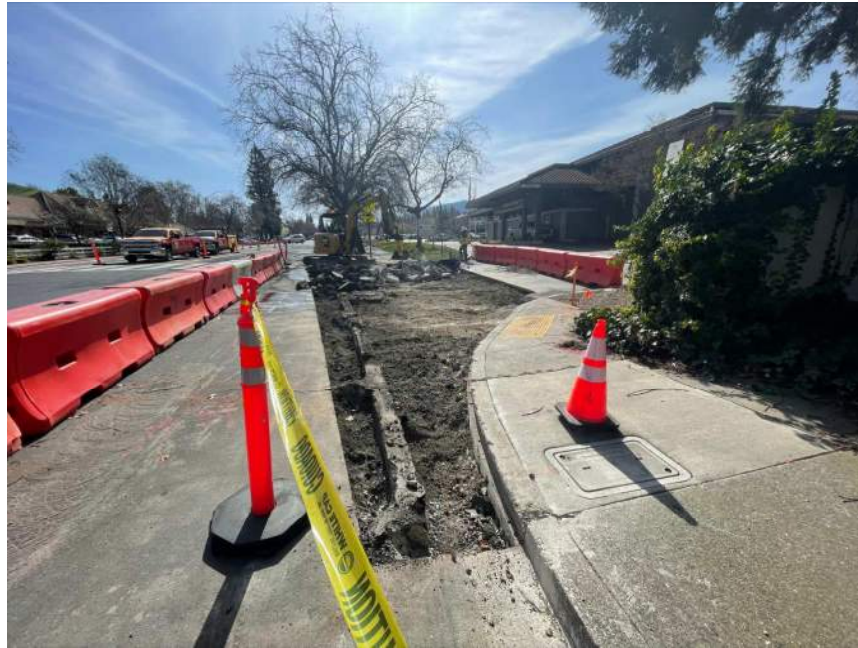
Figure 1. Demolition of existing driveway at Jackson Intersection
