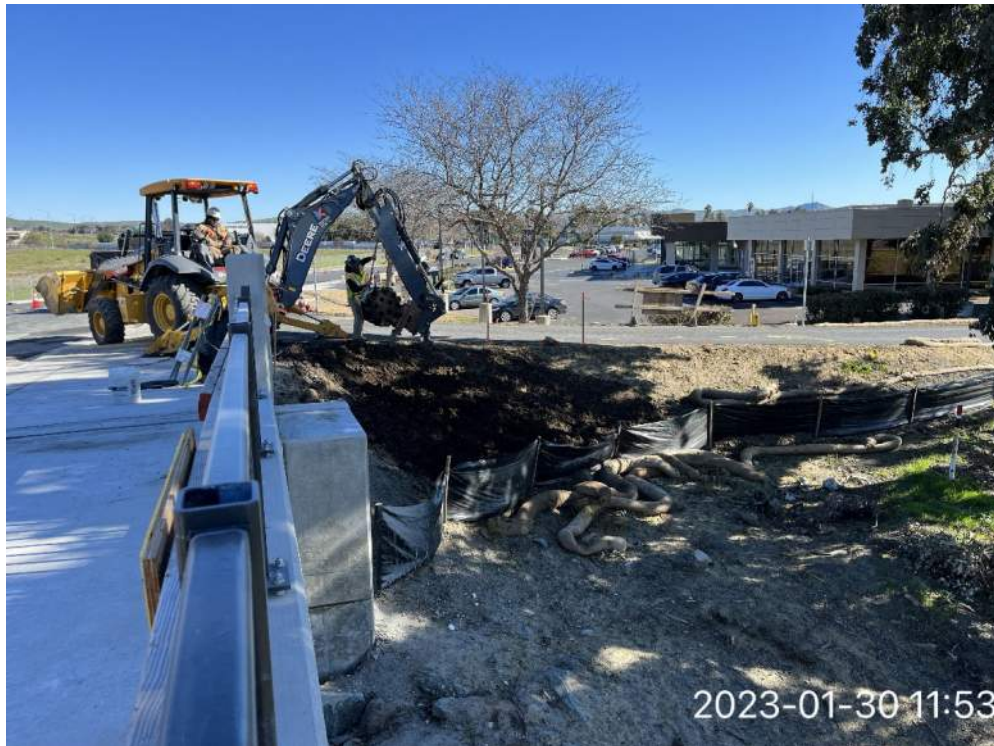
Figure 2 – BCGP Fixing Slope along IHT
