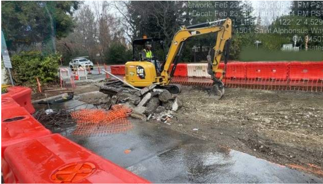
Figure 1. Grading for the future valley gutter and driveway at Jackson Intersection
