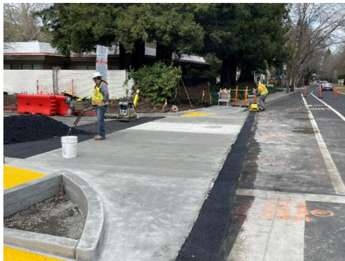
Figure 2. The newly completed driveway and curb ramps at the Jackson Intersection
