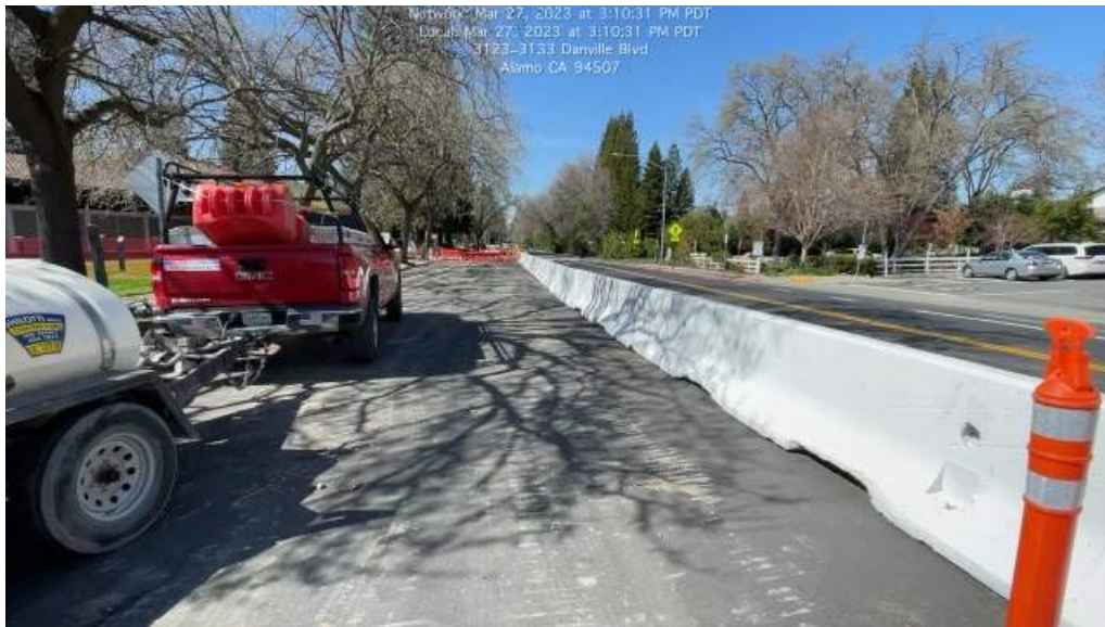
Figure 2. The temporary concrete barriers placed to delineate the work zone.
