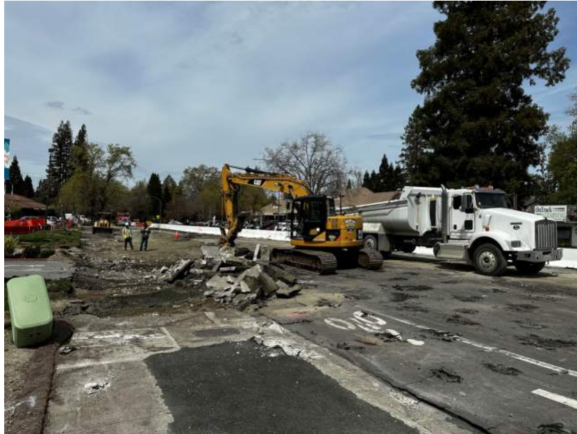
Figure 1. Demolition of the existing roadway.
