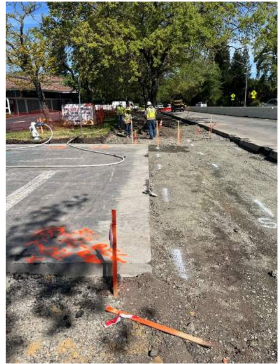
Figure 2. Survey Layout of future roadway improvements
