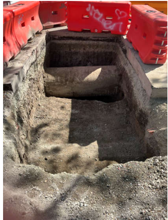
Figure 2. Preparation for Drainage Connection
