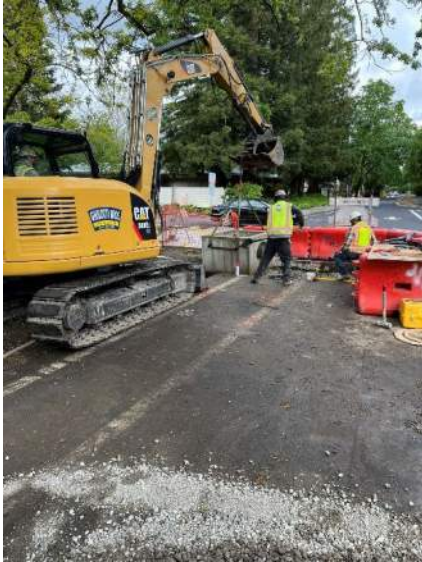
Figure 1. Storm Drain Box Installation
