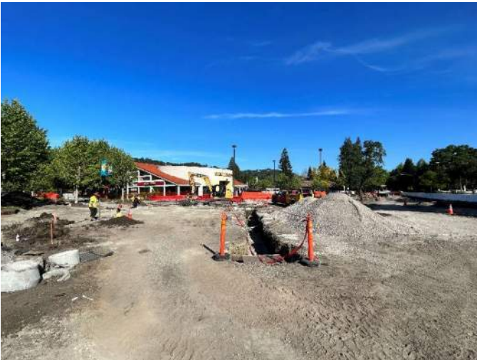
Figure 1. Storm Drain Installation @ new Alamo Plaza Entrance
