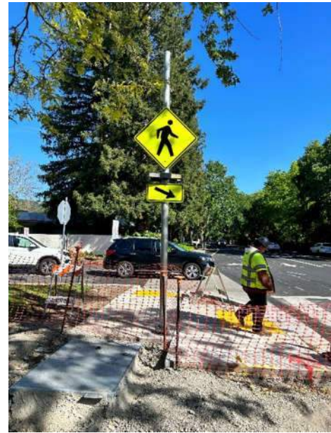
Figure 2. Re-installed Pedestrian Flashing Xing at Jackson Way
