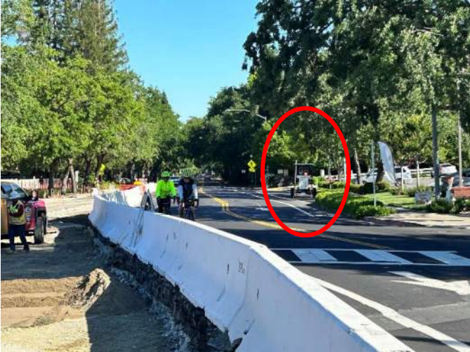
Figure 1. - Construction Area speed enforcement
