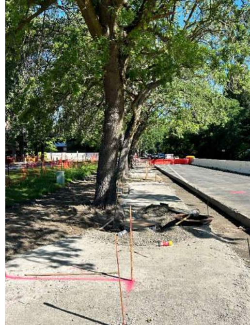
Figure 2. - Subgrade preparation for new sidewalk
