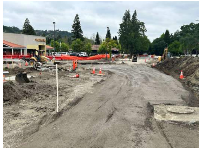
Figure 2. - Subgrade preparation for new roadway
