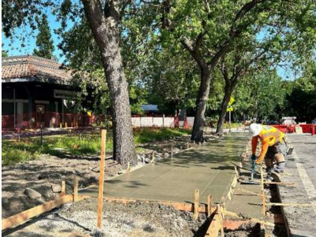
Figure 1. - Sidewalk Finishing
