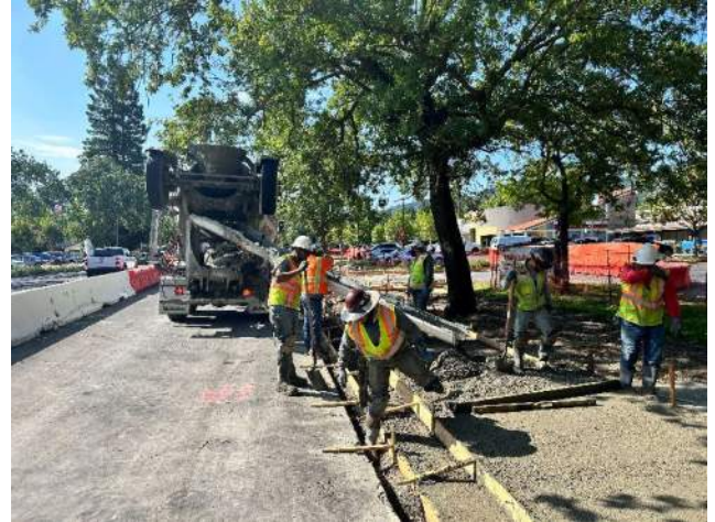
Figure 2. - Concrete Placement for west sidewalk
