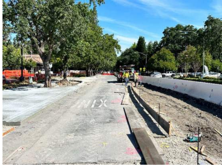
Figure 2. - New Sidewalk and forming Island
