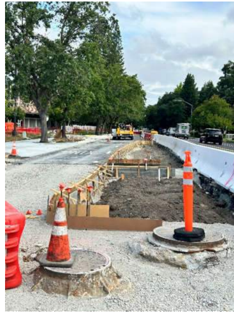
Figure 2. - Center Median formwork
