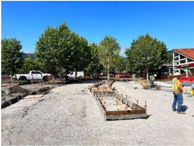
Figure 1. - Alamo Plaza Entrance formwork
