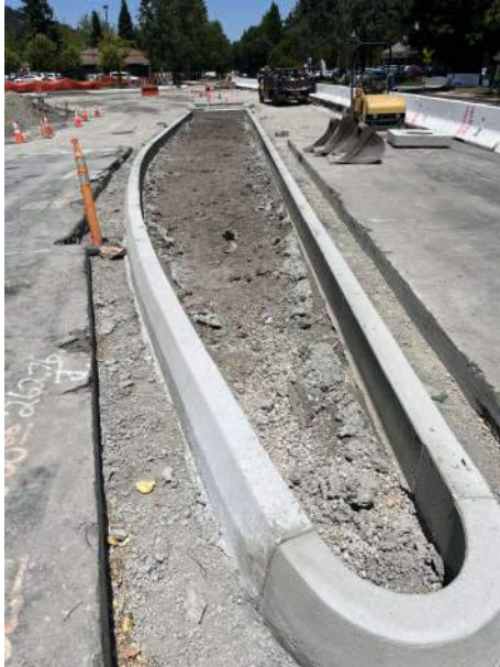
Figure 1. - Center Median Formwork Stripped
