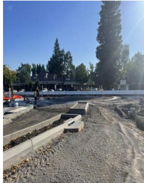
Figure 2. - Round about installation
