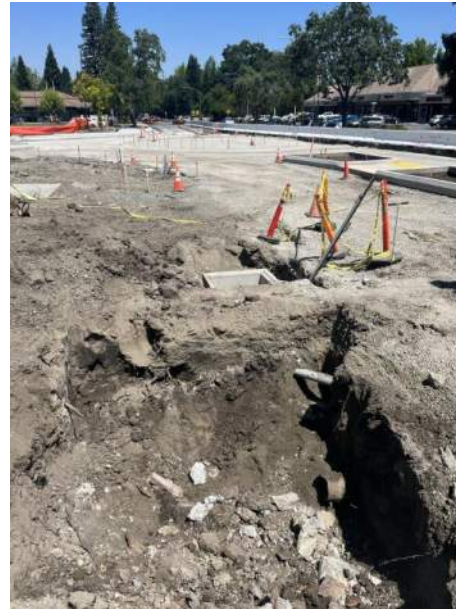
Figure 2. - Storm Drain Installation
