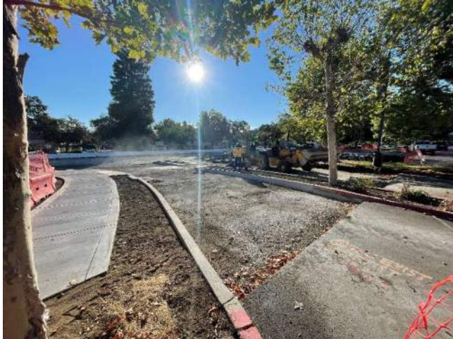
Figure 1. - Alamo Plaza Entrance Subgrade
