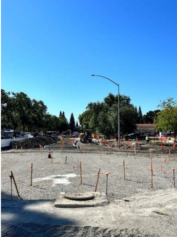
Figure 1. - Roundabout Staking
