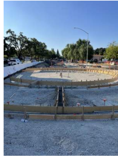
Fig. 2. - Round About Formwork
