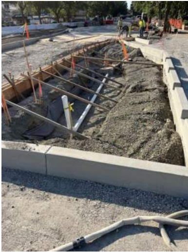
Figure 1. - Curb Formwork/Bioretention Facility
