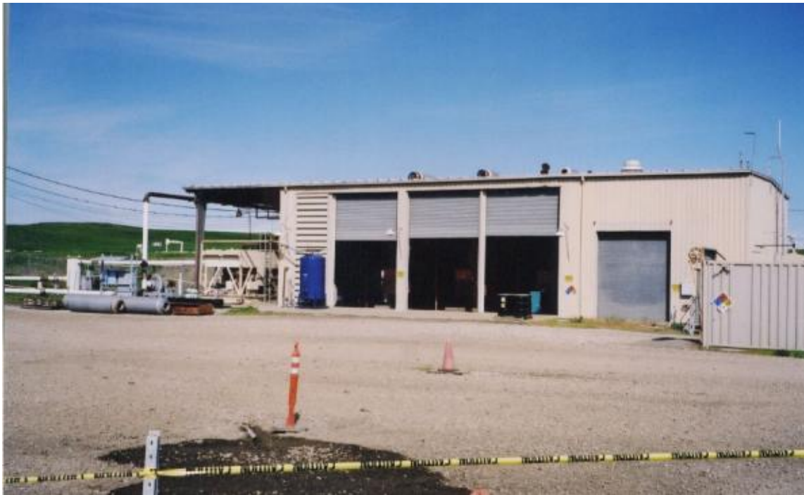
Figure 10-2. LFG Power Plant. Located in WCCSL Area A, this plant generates about 3 megawatts of electricity from LFG, enough to power about 3,000 homes.
