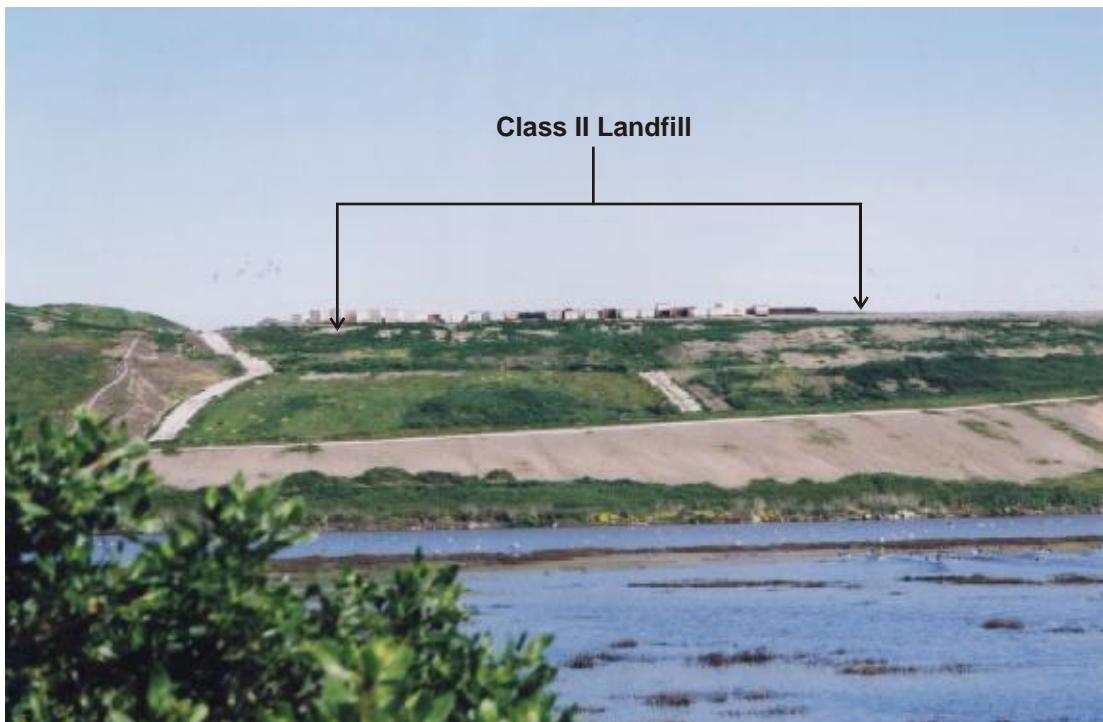
Figure 5-4 Landfill Seismic Displacements. The Southern area of the Class II landfill shown here is less stable than other areas under certain seismic conditions. A detailed earthquake response plan will be developed by the Applicant (Control Measure 5.7 (d))
