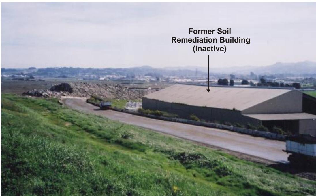
Figure 5-2 Settlement of the Former Soil Remediaton Building. This building would be rehabilitated and expanded for the proposed WRC. It is located on fill which has experienced substantial differential settlement since it was constructed in 1996.
